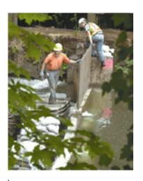
Erich Rabe (left) and Nick Bales of K.T. Contracting Company Inc. build a temporary dam under the Commercial Street bridge for Pringle Creek. The dam will divert water from the construction area so that engineers can build a new weir and fish ladder under the bridge.
